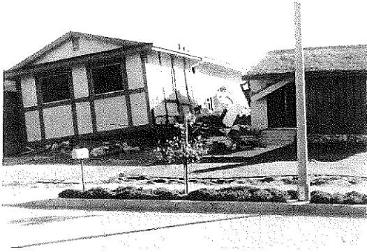
Condition 1: Collapse, partial collapse, or moved off foundation. Post as Closed.
